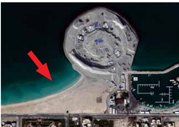
Figure 9. Interruptions in natural sediment drift (in this case increased deposition of sediments on the left side of the structure) can modify the natural shape of a shoreline. The red arrow indicates the direction of predominant wave action (Source: 'Umm Suqeim 2 Harbor.' 25°09'08.01' N and 55°11'50.46' E. (Source: Google Earth, 23rd February 2011).
