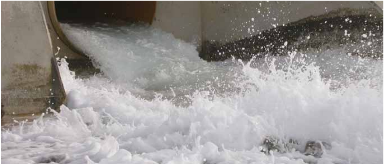
Thermal hypersaline effluent from a power/desalination plant in Abu Dhabi is being discharged into the sea (2009). Credit: Edwin Grandcourt
