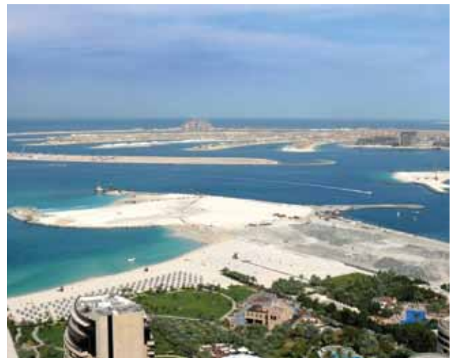
The Gulf region contains the largest man made islands in the world; this poses numerous environmental challenges (Palm Jumeirah island, Dubai, UAE, 2007). Credit: Imre Solt, Dubai Constructions Update ( www.imresolt.com )
