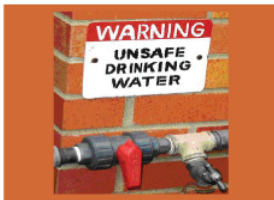
Unsafe Drinking Water
