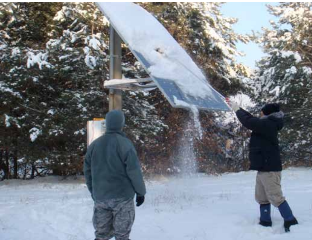
Clearing the build-up of snow from a solar panel at PS31.
