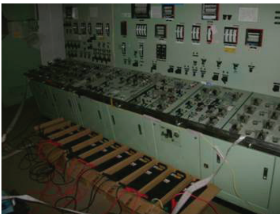
FIGURE 8 Car Batteries Powering Control Panel Source: TEPCO.
