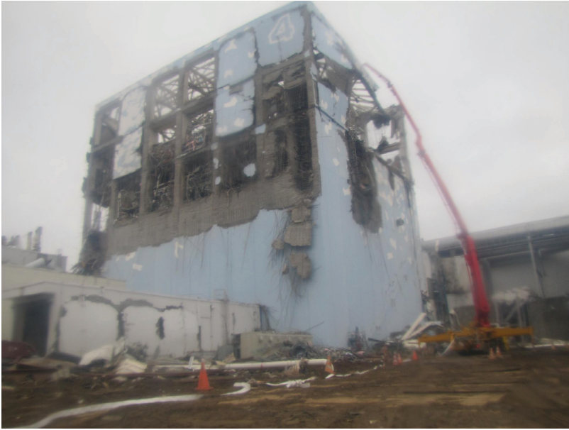
FIGURE 11 “Kirin” Injecting Water into Reactor 4, March 22, 2011 Source: TEPCO ( http://www.tepco.co.jp/en/nu/fukushima-np/review/review1_2-e.html ).
