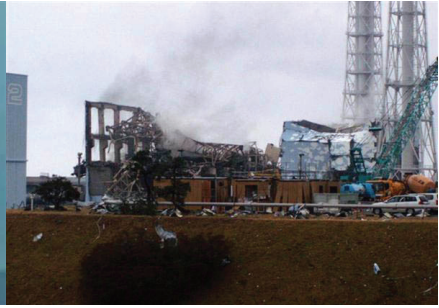
FIGURE 3 Aftermath at Fukushima Dai-Ichi plant Reactor 3 Source: TEPCO.
