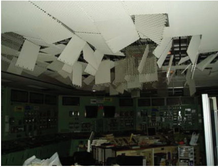
FIGURE 6 Central Control Room after Reactor 1 Explosion Source: TEPCO.
