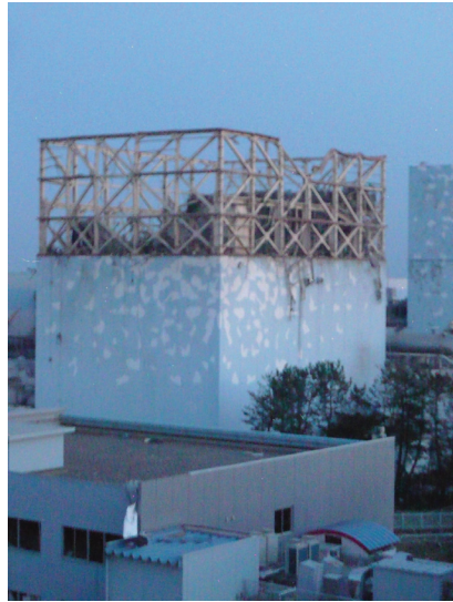
FIGURE 7 Aftermath of Reactor 1 Explosion Source: TEPCO.
