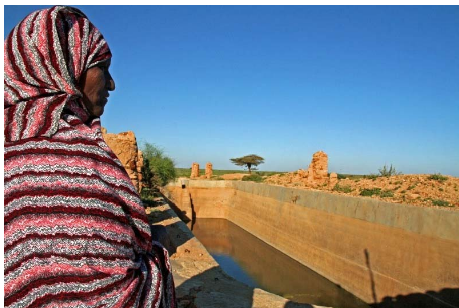
Sarahaa Malmud Muhumed next to an Oxfam-built birkhad , a protected pond for collecting rainwater to use during the long dry season, Harshin, Somali region. Credit: Oxfam/Maite Alvarez
