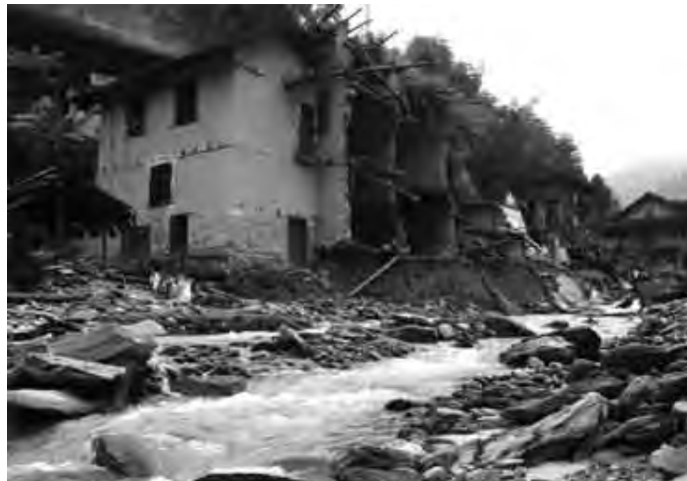
Recent violent floods have caused a rapid rise in the river taking away rows of houses in Xinshao, Hunan Province, China. Photo: © 2005 Greenpeace/Hu Wei
