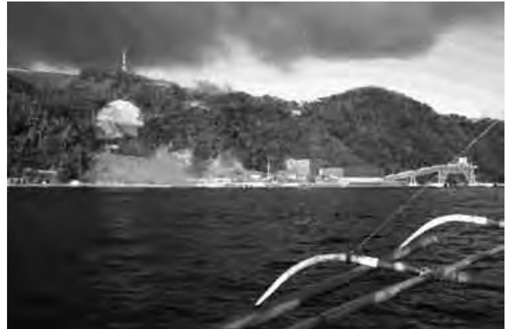
A landslide at the RapuRapu mine: part of the extensive damage that occurred to buildings and the environment after the November 2006 typhoon.
