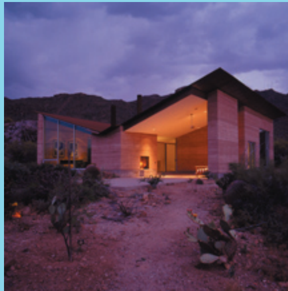
The Tucson Mountain House with rammed earth walls designed by Rick Joy.
