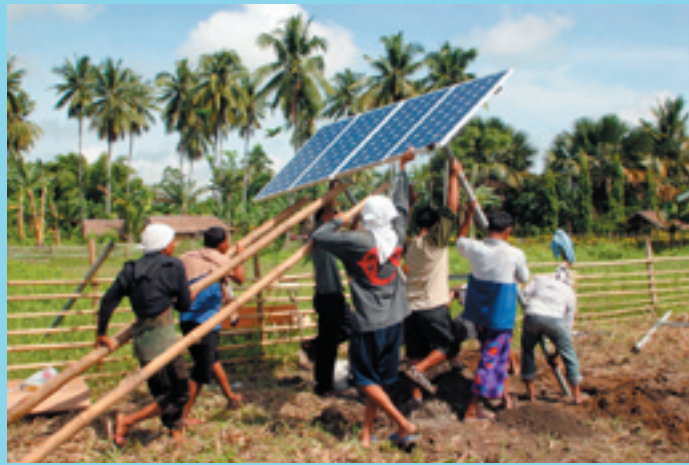
Villagers erect a solar photovoltaic panel in Mindanao, Philippines.
