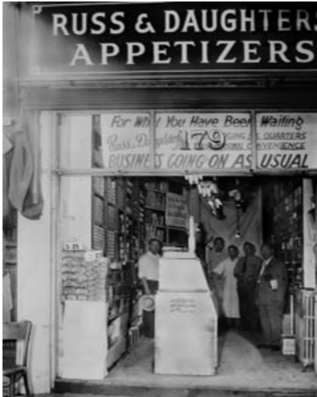
Russ & Daughters' landmark store on New York City's lower east side. Established in 1914, the business has been run by four generations of the Russ family. (Photo courtesy of russanddaughters.com)
