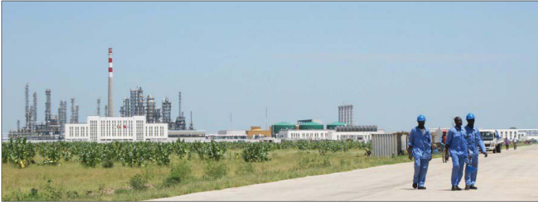
Figure 4: Workers Leaving the Refinery in Djarmaya
