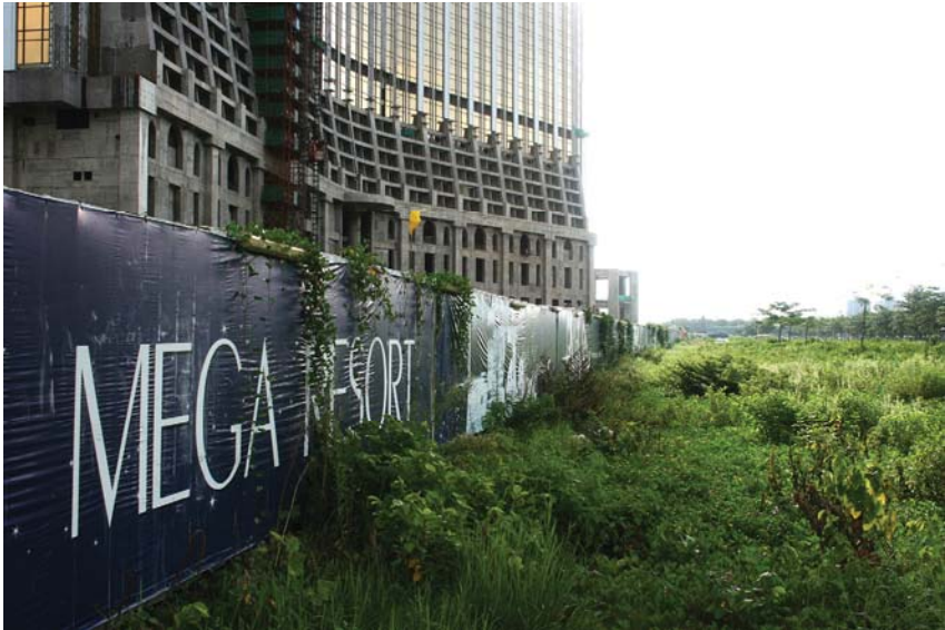
Figure 5: Casino Construction on Hold at Macau's Cotai Reclamation
