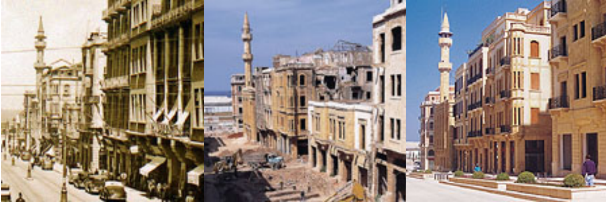
Image 7. Example of Solidere's restoration works: Restored quarter in Beirut's Central District
