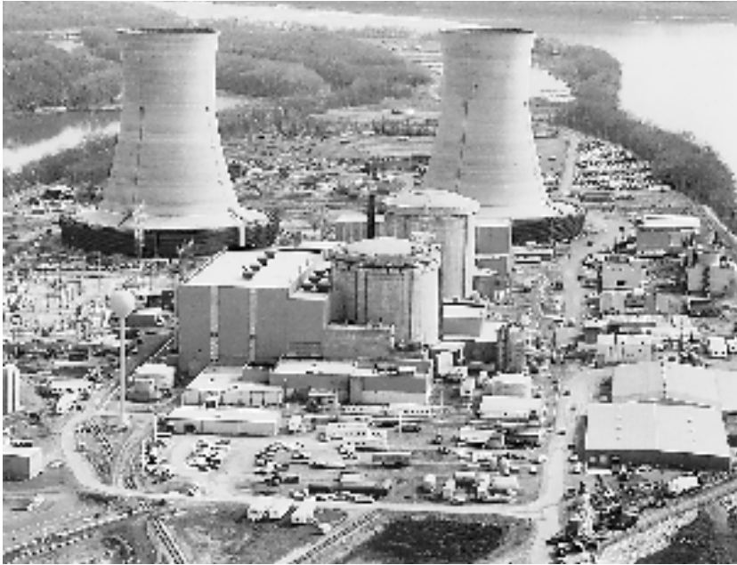
FIGURE 6.1. The Three Mile Island (tmi) power plant ten miles south of Harrisburg, Pennsylvania, showing the two cylindrical containment buildings ( center ) and two of the cooling towers ( background ) of the plant. The history of TMI is described in the newspaper article reproduced in figure 6.2.
