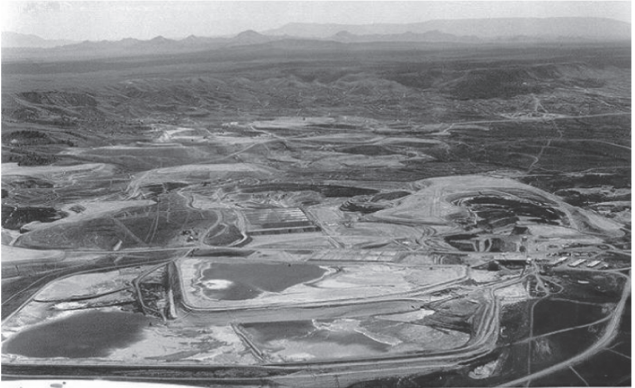
The Umetco Minerals Corporation mill in Gas Hills, Wyoming, ceased operation in 1984 and was decommissioned in 1990. This picture depicts the site before its reclamation under the Uranium Mill Tailings Radiation Control Act (UMTRCA).
